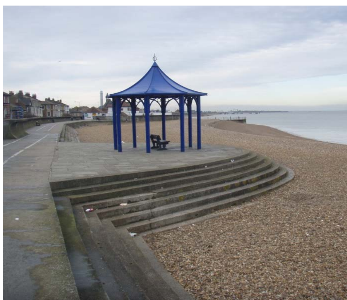
Concrete Stepped Revetment and beach at Sheerness
