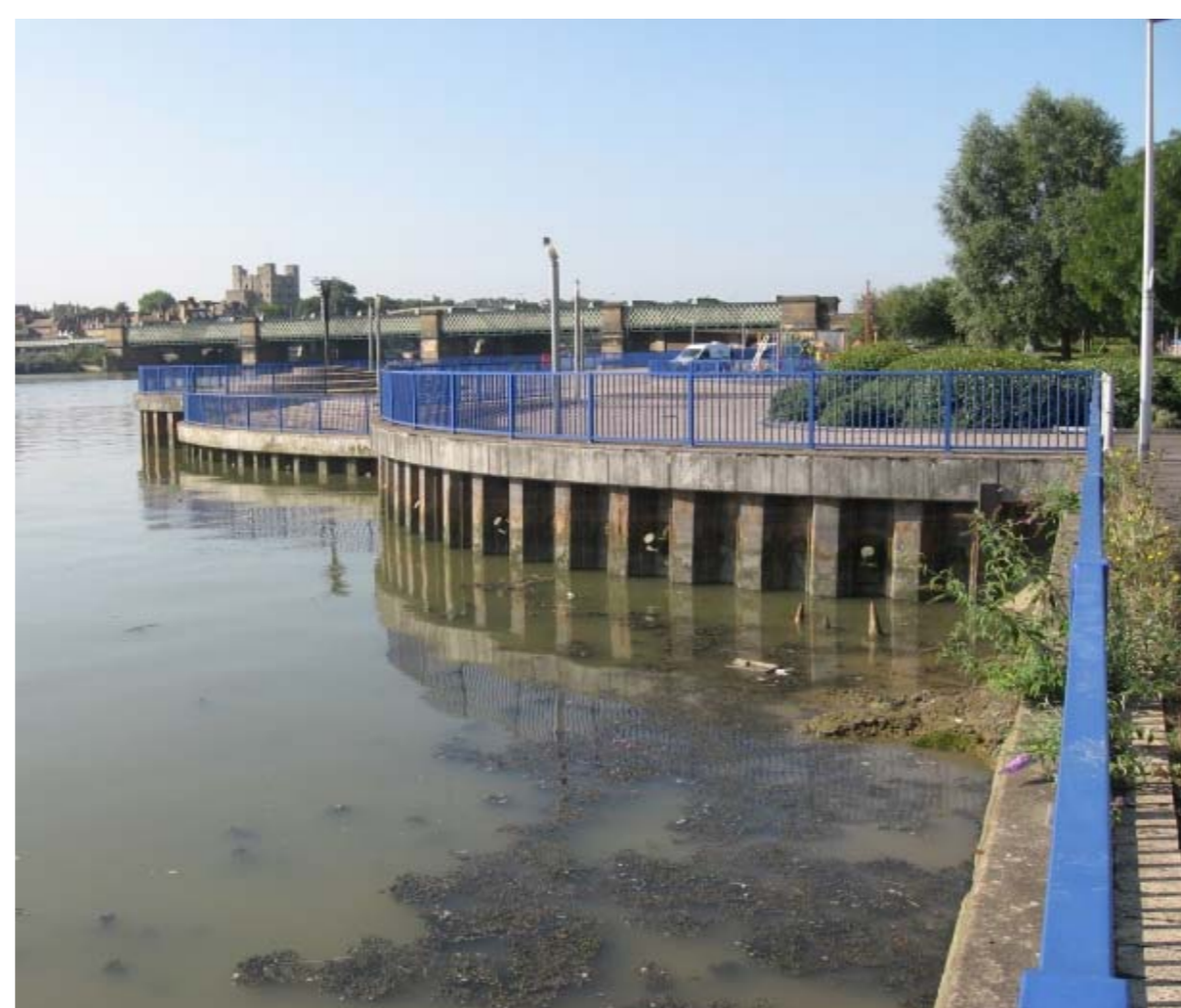
Sheet piled wall along Strood Canal
